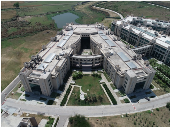
A and B blocks where Department of Physics Labs and offices are located
